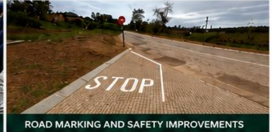
ROAD MARKING AND SAFETY IMPROVEMENTS
